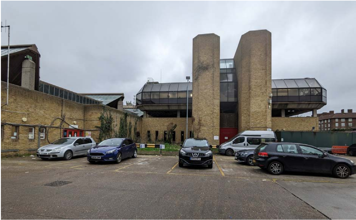
Fig X: Ash Grove bus garage angled stair structures, upper level office and garage roof structure
