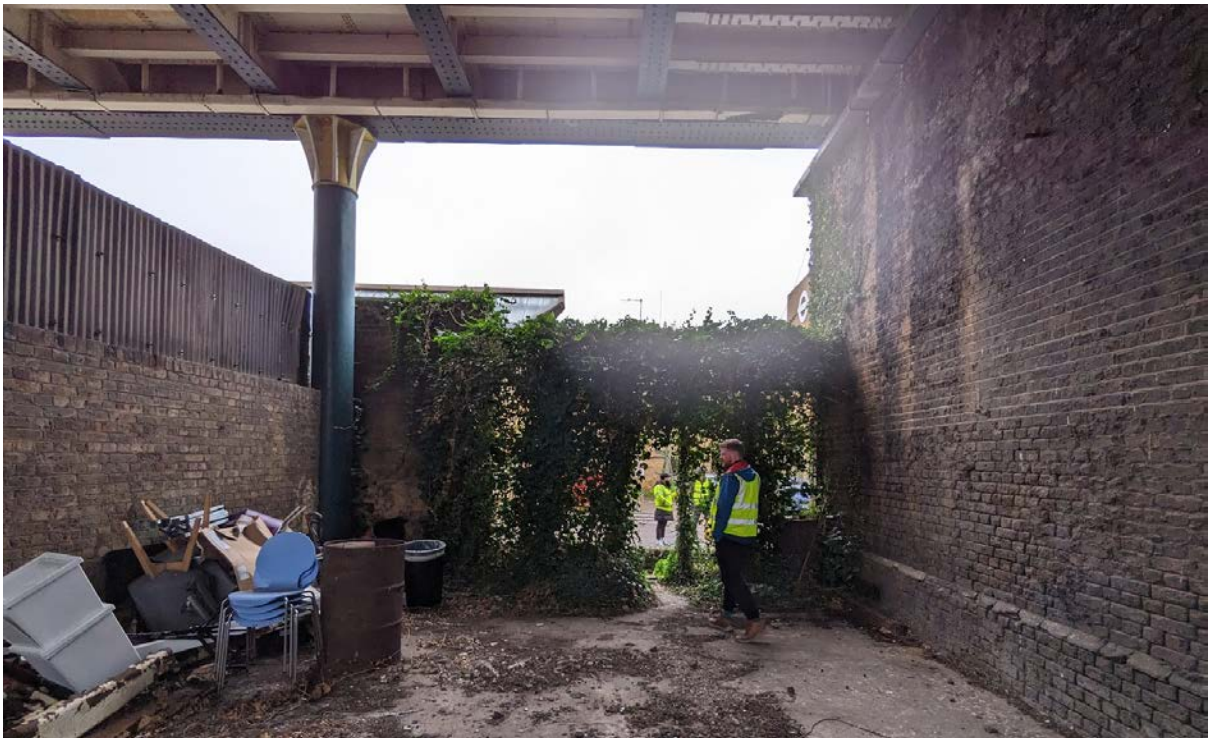
Fig X: unused space underneath the section of railway bridging over Ash Grove, including original column.
