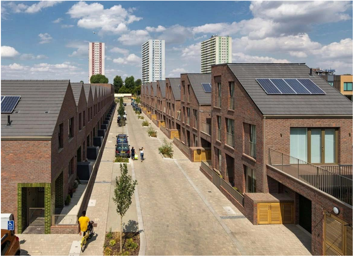
Fig X: pedestrian routes, parking/loading bays and vehicles routes are separated by different surface treatments and planting at Dujardin Mews by KCA architects (photograph Tim Crocker) 48
