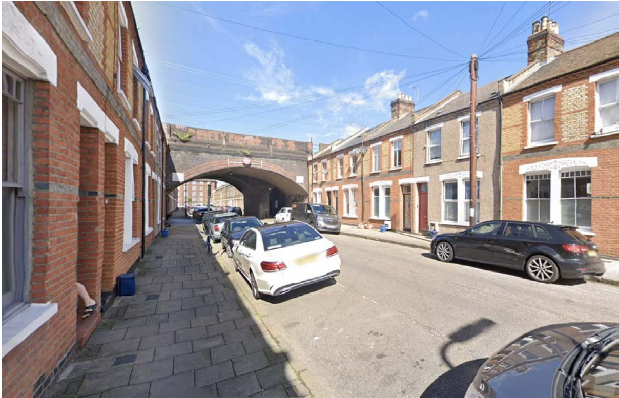
Fig X: Beck Road terraced houses and railway arch
