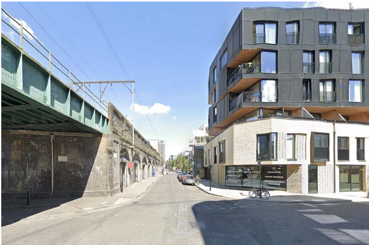
Fig X: Mentmore Terrace in London Fields, an example showing the potential relationship between converted railway arches and taller new buildings
