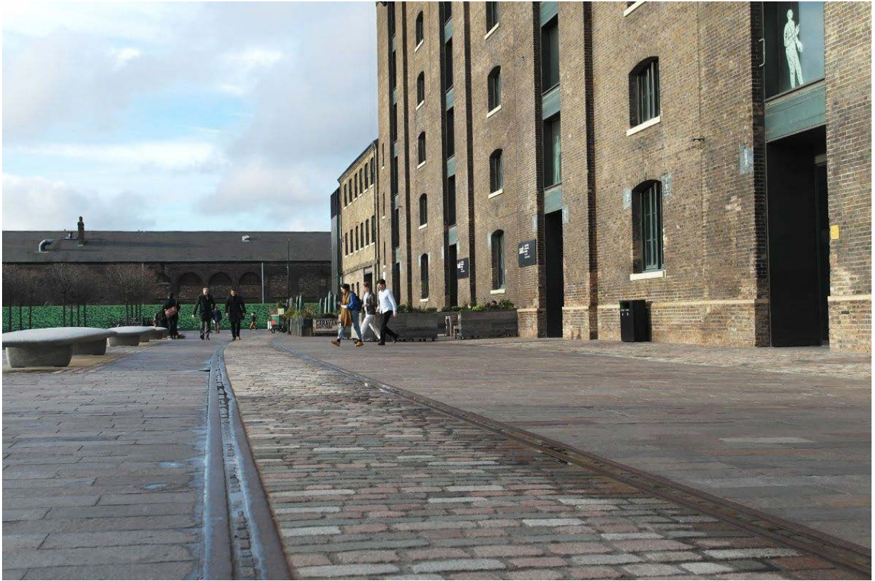
Fig X: Tram/rail lines in Granary Square are a good example of transport infrastructure incorporated into the design of a new public space 19
