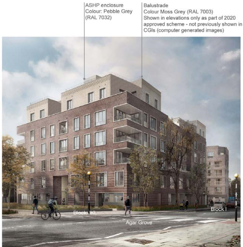
Fig X: showing proposed ASHP enclosures on the roof of proposed buildings at Agar Grove, London 76
