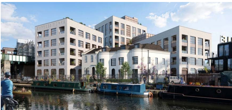
Fig X: Empress works (on the other side of Regent's Canal to the bus garage) is an example of how new buildings can respond to an existing heritage building, while building taller than the immediate and surrounding area 21 .
